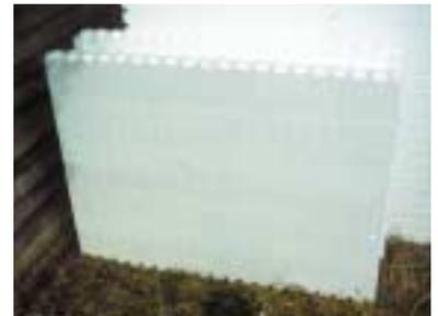
Figure 1: The blocks mesh together perfectly and do not require mortar or grout.
